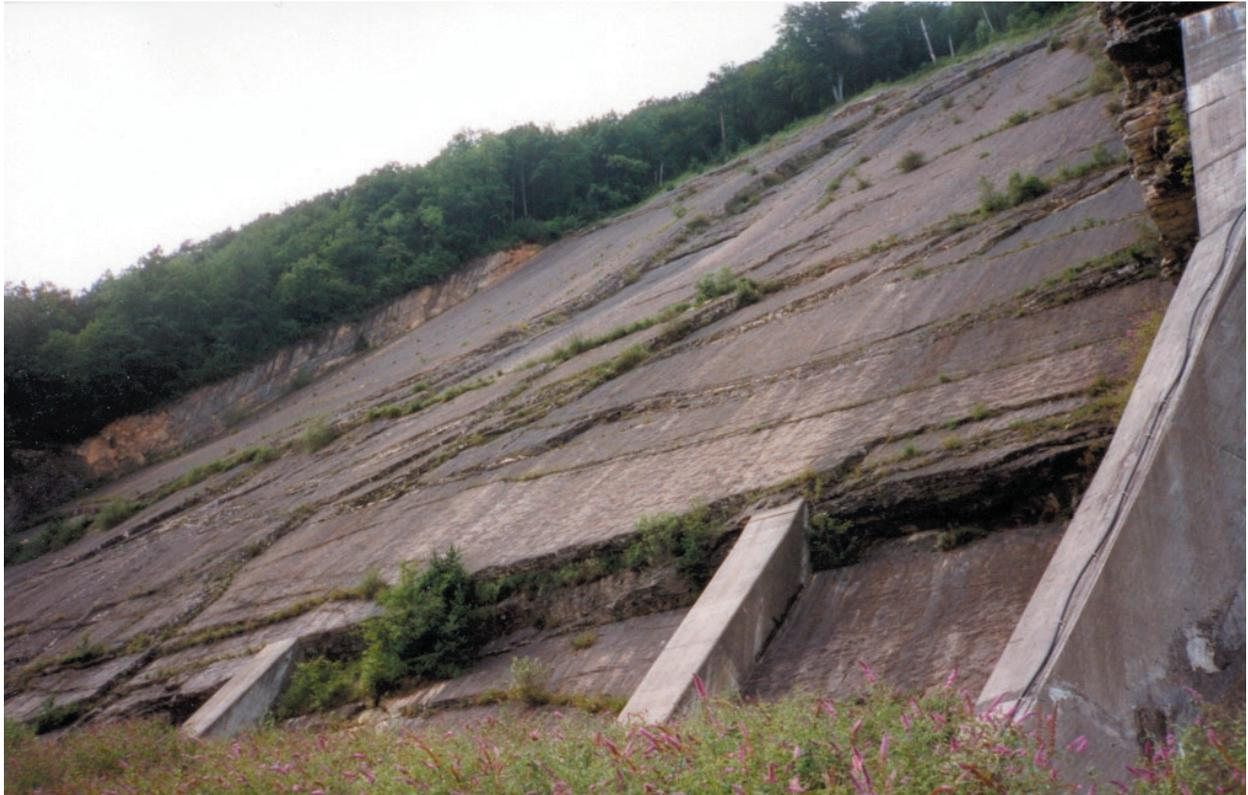
Fig. 5.1.9 : Pillar supporting the foot of a dip-slope limestone series in the Eichwald quarry (west of Brunnen, Canton of Luzern). Photo Parriaux.
