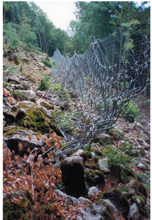
Fig. 5.1.5 : Geobrugg net for retaining blocks. Photos Geobrugg AG.
