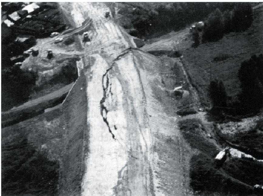
b) General view of an embankment after a circular rupture.
